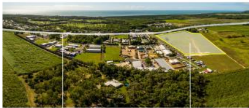
Captain Cook Highway Connecting Cairns & Port Douglas
