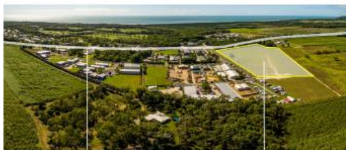
Captain Cook Highway Connecting Cairns & Port Douglas
